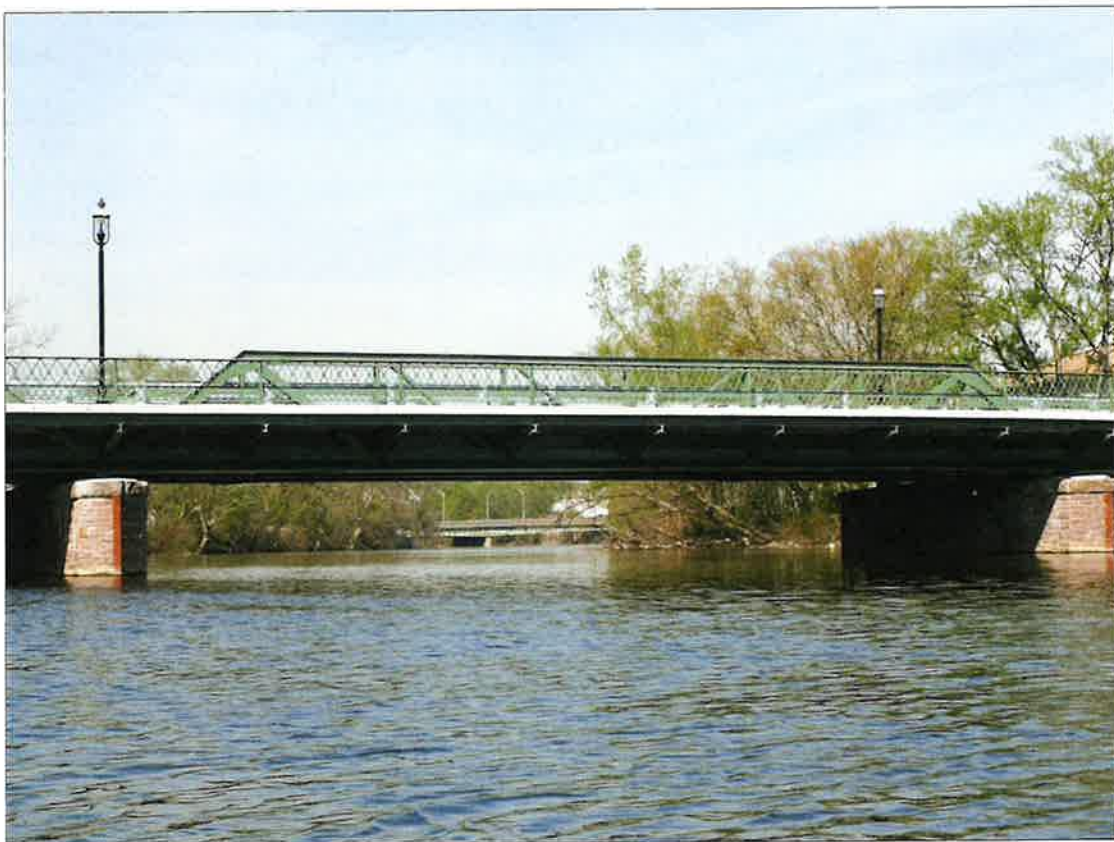
Figure 7. The Passaic River and the Hillery Street Bridge near Woodland Park, New Jersey (2009). The location of this bridge is marked in Figure 2.
