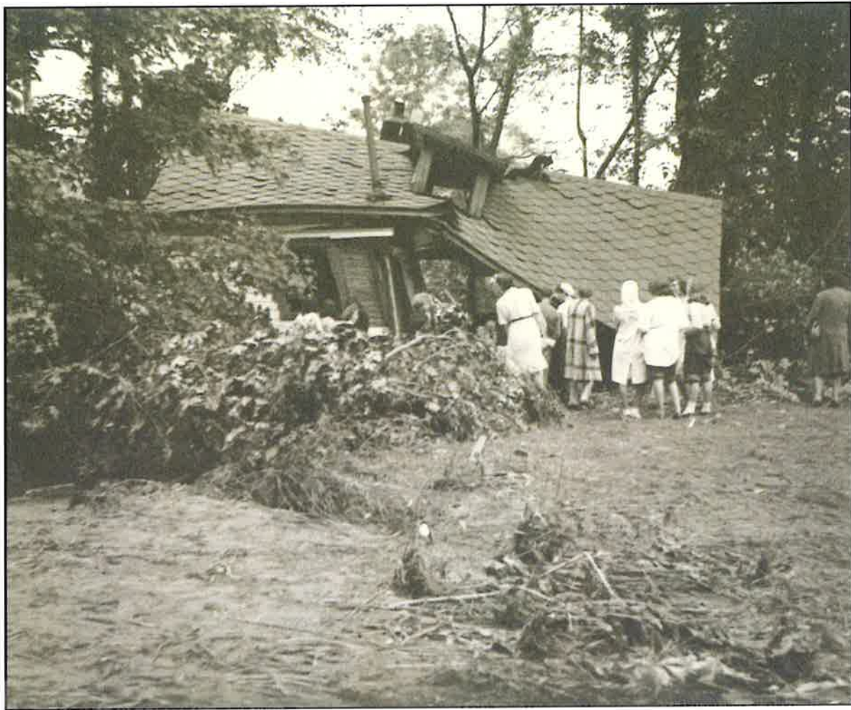
Figure 19. The Riker family house on Cedar Grove Road in Little Falls, NJ after it had been destroyed by the Peckman River flood of 1945. The house was split down the middle and collapsed. The house was washed from its foundation and collapsed, killing a woman who lived there. Courtesy of the Little Falls Historical Society. Photographed July 22, 1945.
