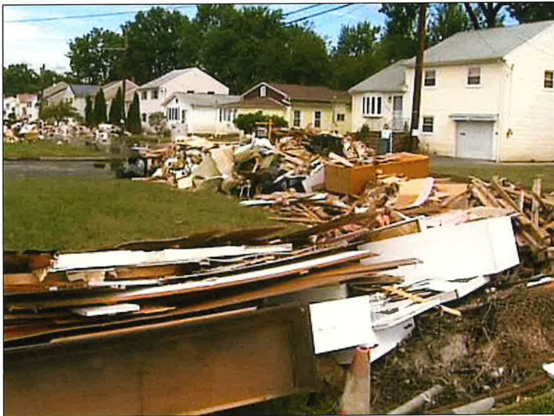
Figure 51. Flood damage in Little Falls after Hurricane Irene (2011).
