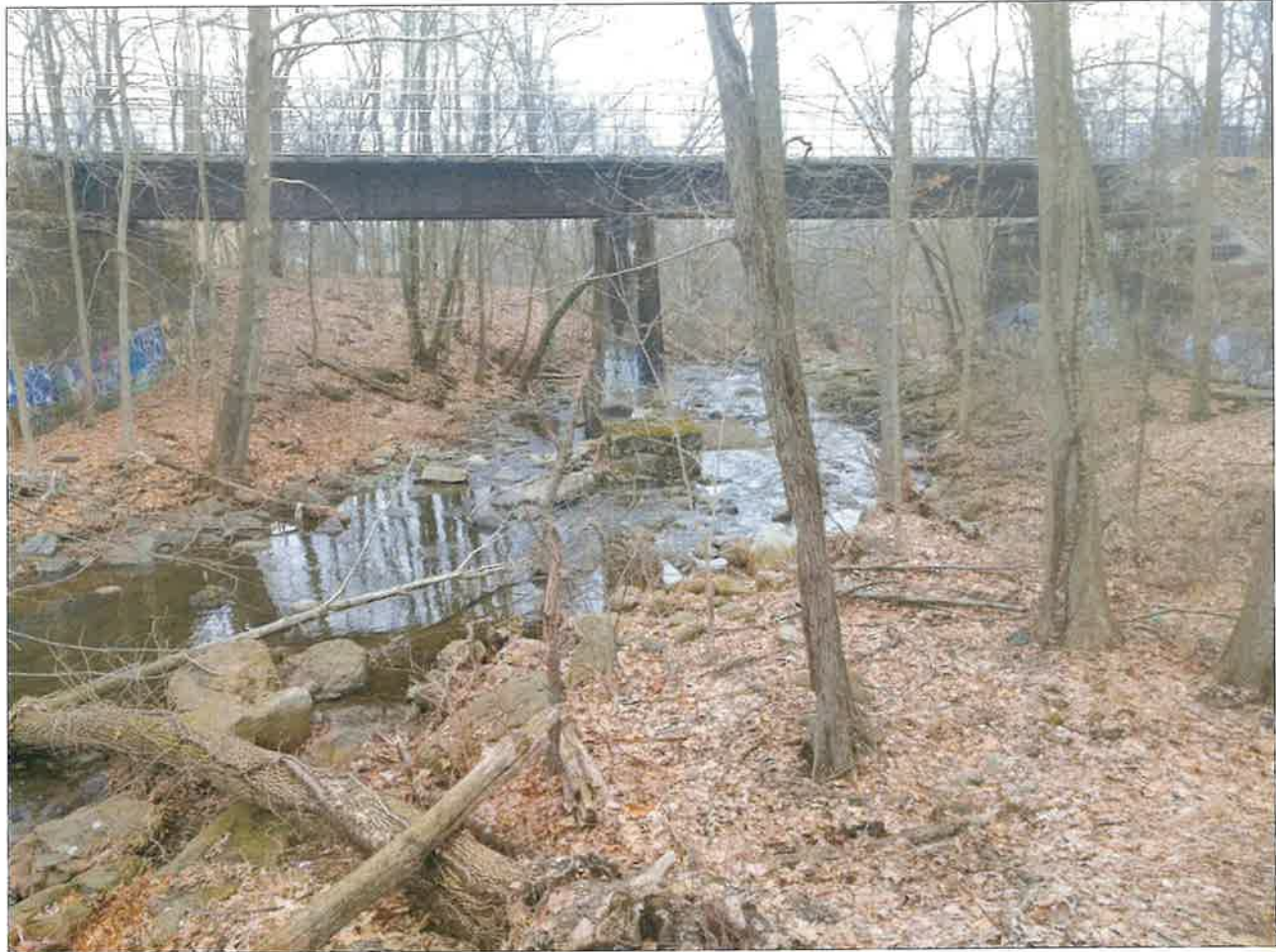
Figure 6. The Peckman River at the West Essex Trail crossing (2018).
