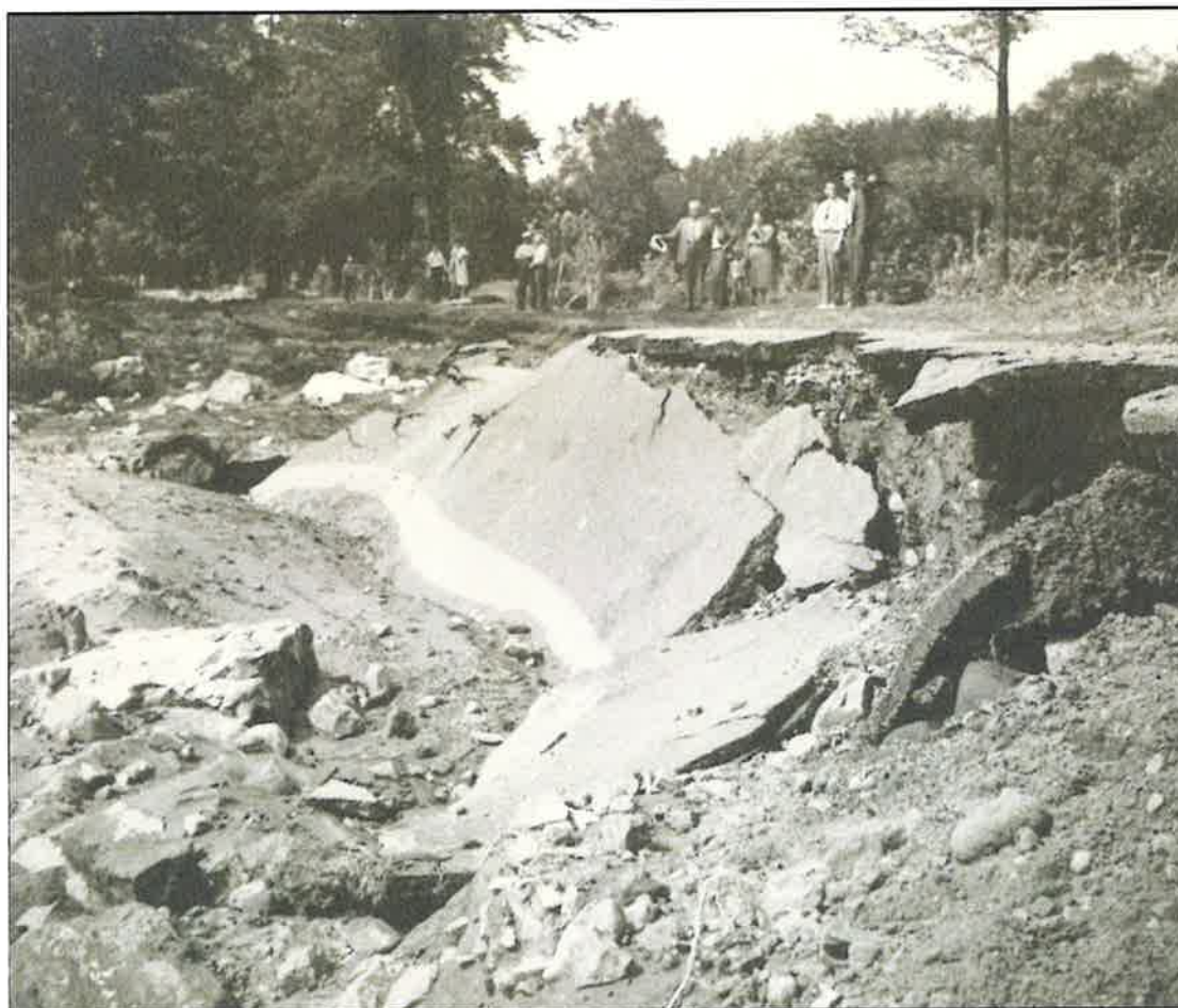
Figure 17. A road that was washed out in Little Falls during the 1945 flood. Photo courtesy of the Little Falls Historical Society. Photographed July 22, 1945.
