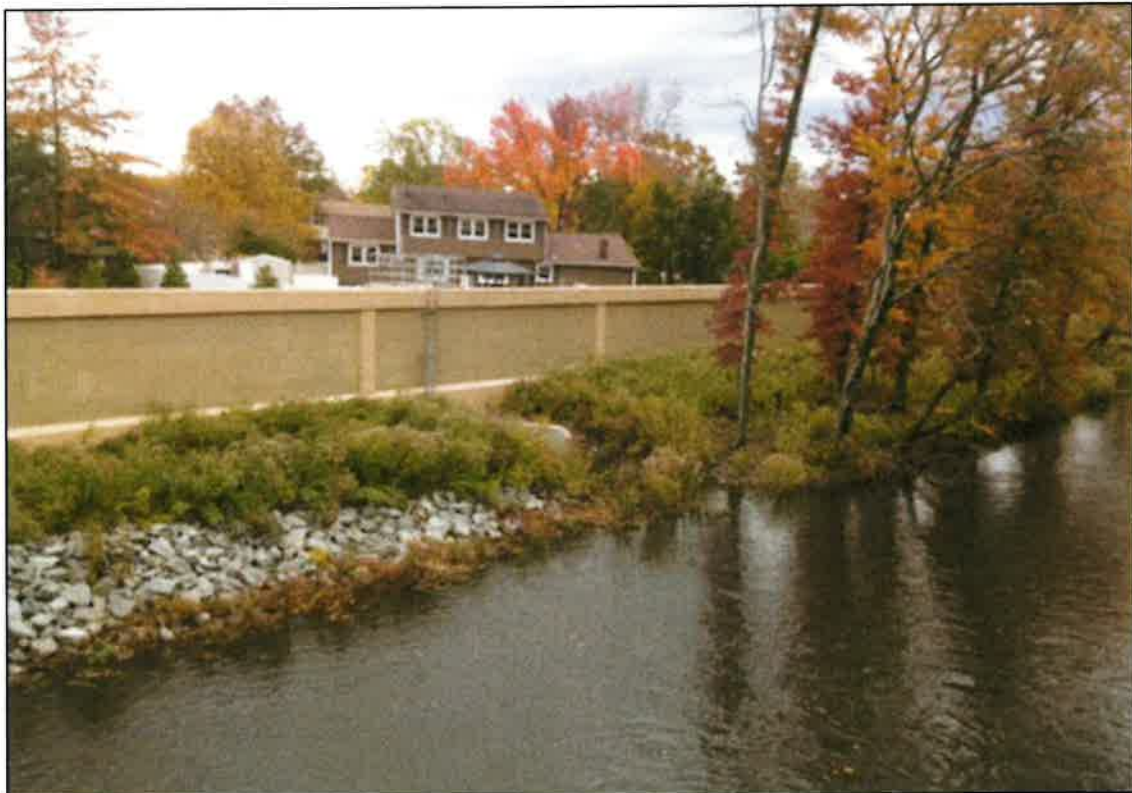
Figure 39. An example of a permanent floodwall in Middlesex, New Jersey.
