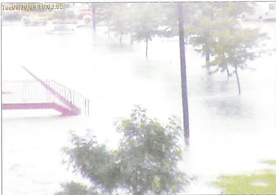
Figure 31. Pedestrian bridge over Great Notch Brook pictured in previous figure during the June 30, 2009 storm.
