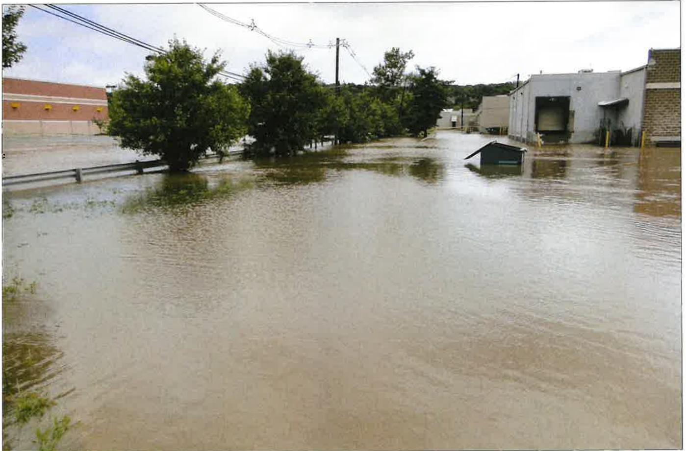
Figure 35. Flooded commercial area in Woodland Park, New Jersey.
