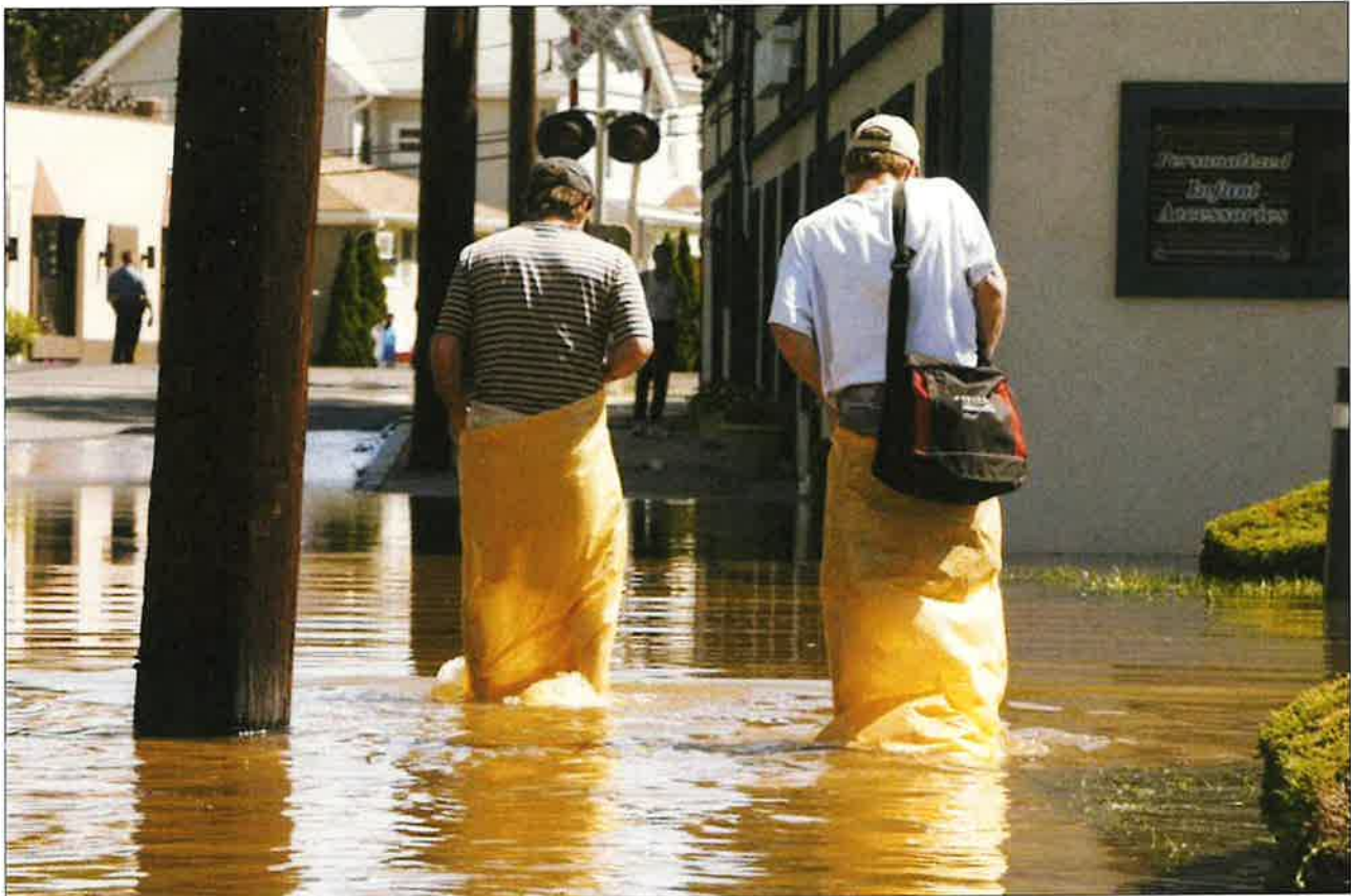
Figure 22. Flood damage in Little Falls, New Jersey after Hurricane Irene (2011).
